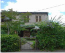
carlton north station street carlton north station street 467
