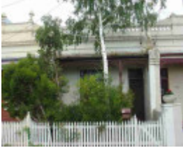
carlton north station street carlton north station street 468
