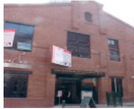
Former Angliss Stables May 2003
