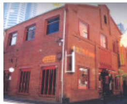
Former Stables as Restaurant
