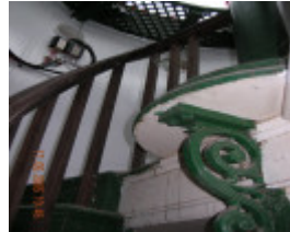
WEST CHANNEL PILE LIGHT SOHE 2008
