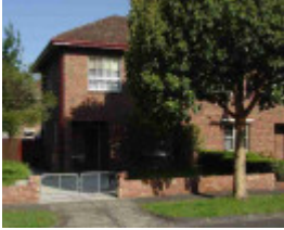
burnley tudor street burnley tudor street 5
