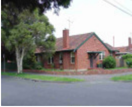
burnley tudor street burnley tudor street 30
