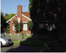
burnley tudor street burnley tudor street 33
