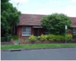
burnley tudor street burnley tudor street 36
