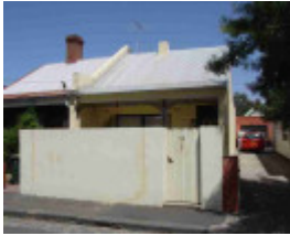
richmond tyson street richmond tyson street 16
