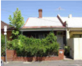
richmond tyson street richmond tyson street 18
