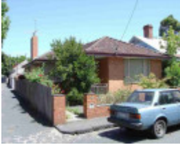
richmond tyson street richmond tyson street 20
