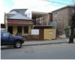
fitzroy kerr street fitzroy kerr street 107-109
