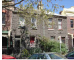
Fitzroy Kerr Street 110-112.JPG
