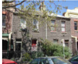
Fitzroy Kerr Street 110-112.JPG
