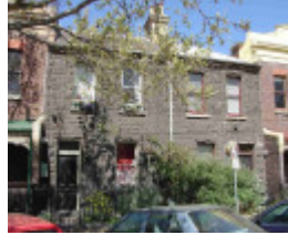
Fitzroy Kerr Street 110-112.JPG
