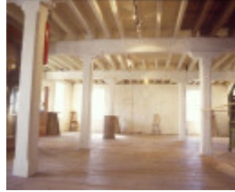
h00389 portarlington mill turner crt portarlington first floor construction she project 2003
