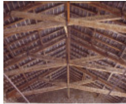
h00389 portarlington mill turner crt portarlington scissor beam construction under roof she project 2003
