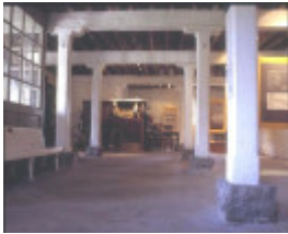
h00389 portarlington mill turner crt portarlington ground floor she project 2003
