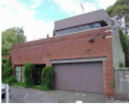
richmond verity street richmond verity street 13
