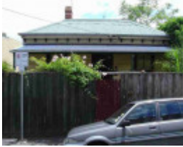
richmond verity street richmond verity street 14
