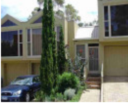
richmond verity street richmond verity street 18
