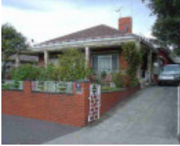
clifton hill heidelberg road clifton hill heidelberg road 111
