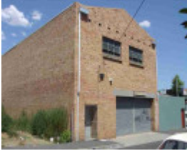
richmond waverley street richmond waverley street 33
