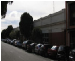
113 Wellington Street - rear view from Cambridge Street
