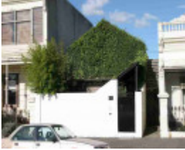
princes hill wilson street princes hill wilson street 54
