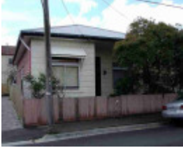
burnley survey street burnley survey street 1
