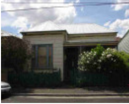
burnley survey street burnley survey street 3
