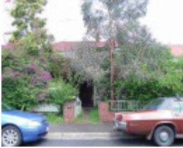
burnley survey street burnley survey street 4
