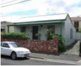
burnley survey street burnley survey street 5
