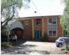
richmond waltham place richmond waltham place 9
