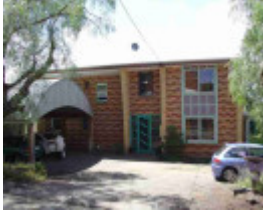
richmond waltham place richmond waltham place 9
