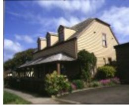
1 former steampacker hotel front view
