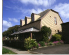
1 former steampacker hotel front view
