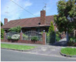
burnley tudor street burnley tudor street 2
