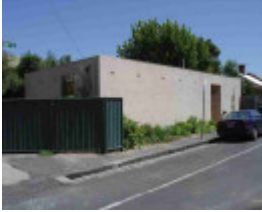
richmond tyson street richmond tyson street 22
