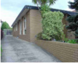
clifton hill heidelberg road clifton hill heidelberg road 107
