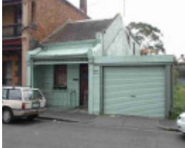
fitzroy argyle street fitzroy argyle street 101-103
