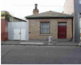
fitzroy argyle street fitzroy argyle street 10
