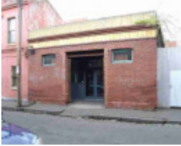
fitzroy argyle street fitzroy argyle street 12
