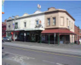
Fitzroy Brunswick Street 403- 411.JPG
