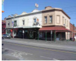
Fitzroy Brunswick Street 403- 411.JPG
