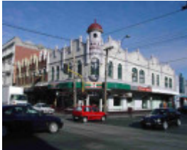
Fitzroy Brunswick Street 287-295.JPG
