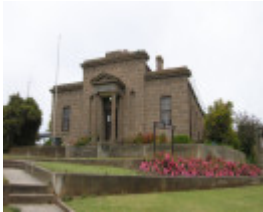
PORTLAND COURT HOUSE SOHE 2008
