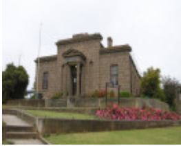
PORTLAND COURT HOUSE SOHE 2008
