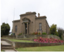
PORTLAND COURT HOUSE SOHE 2008
