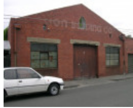
Rear of 45 OGrady Street - A.K.A 28 George Street
