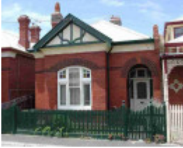
richmond woodlawn street richmond woodlawn street 5
