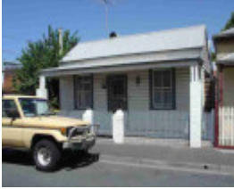
richmond woodlawn street richmond woodlawn street 6
