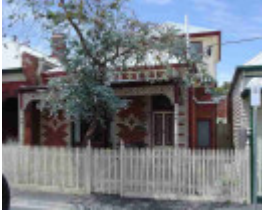
richmond woodlawn street richmond woodlawn street 7
