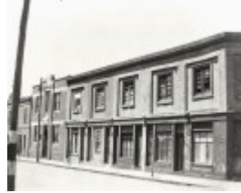
Buildings demolished in slum reclamation
