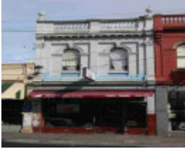
fitzroy brunswick street fitzroy brunswick street 223
