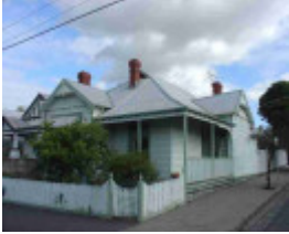
clifton hill fenwick street clifton hill fenwick street 11
