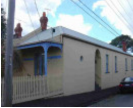
clifton hill fenwick street clifton hill fenwick street 12
