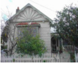
clifton hill fenwick street clifton hill fenwick street 13
