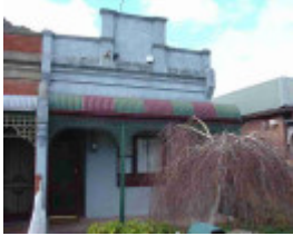
clifton hill fenwick street clifton hill fenwick street 18
