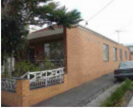
clifton hill fenwick street clifton hill fenwick street 21
