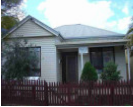
clifton hill fenwick street clifton hill fenwick street 28
